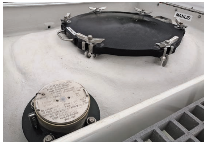
Composite Tank with SRV and manlid
