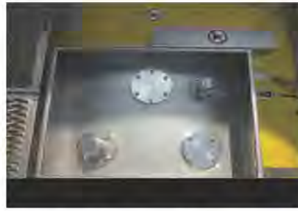
A spill tray housing safety valve provision second safety valve, airline and nozzle for agitator or level gauge
