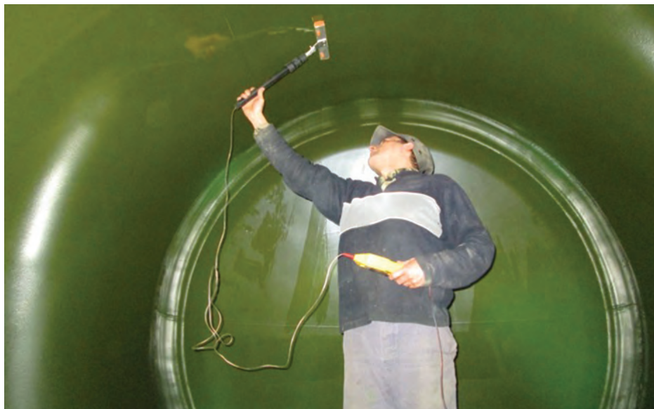
Lithcote has developed a method of curing coatings without the need to first remove the tank container's insulation
